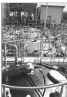
Level measurement in open reservoir with Two-Part System in a sewage treatment plant
