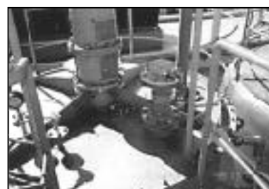
Measurement of an outdoor Sulphuric Acid tank with Compact Transmitter in a chemical plant
